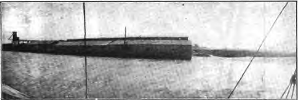
THE SITE OF THE FEDERAL IMMIGRATION STATION AT CHARLESTON.
